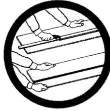
Cutting asbestos-containing wall board by hand
