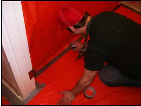
**Worker Constructing Polyethylene Containment**
